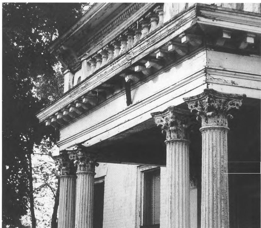
The Columns Alan Havig
